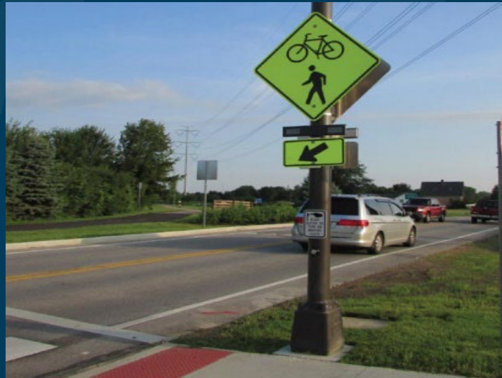
Rectangular Rapid Flashing Beacon (RRFB)
