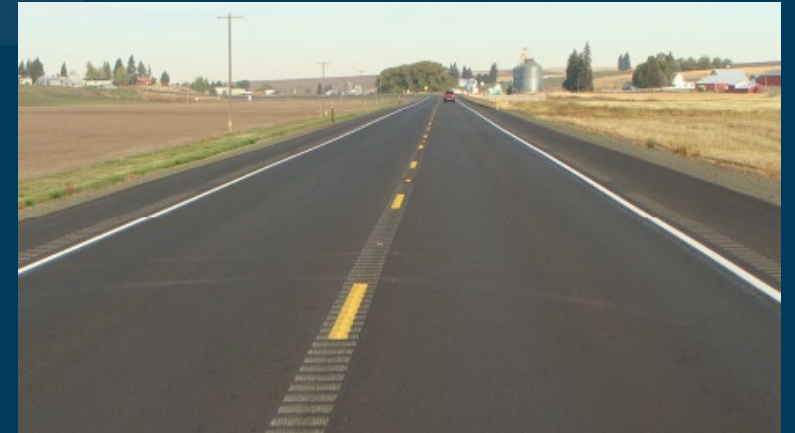
Center Line and Shoulder Rumble Strips
