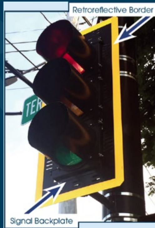
Backplates with Retroreflective Borders
