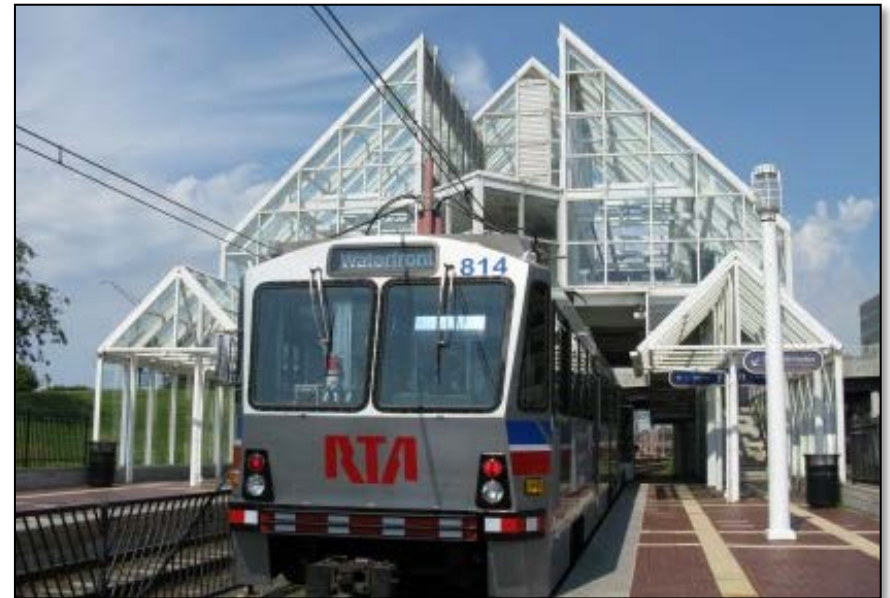
Figure 33: RTA's North Coast Harbor Station
