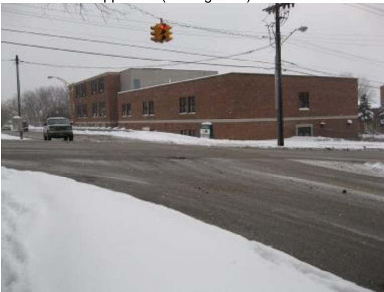
Photo 2 North Approach (looking south)
