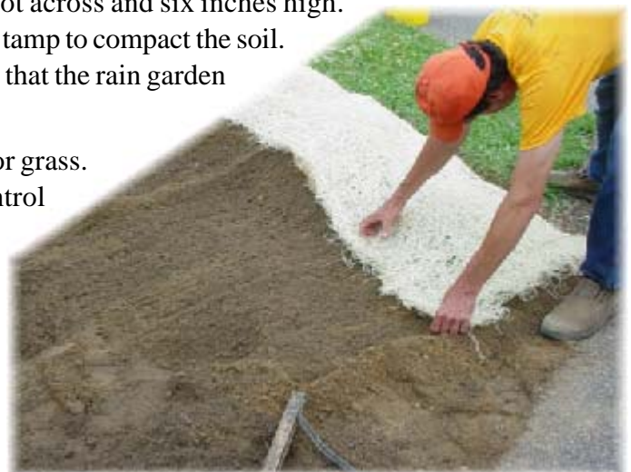
Erosion control matting made of coconut fiber is carefully placed along the berm to prevent erosion on the downhill side of the rain garden.
