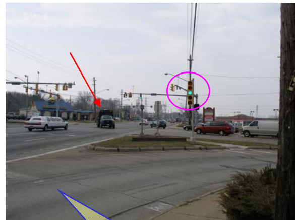
Stop Line is faded, and placed too far from edge of intersection with the main road
