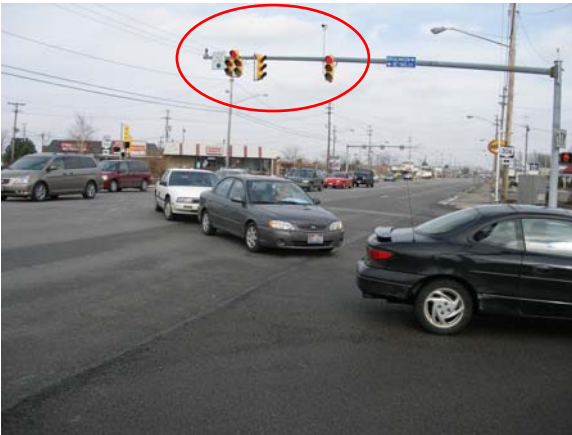
Westbound traffic on US20, turning left onto SR306 southbound during the green interval of the exclusive left turn phase, slows down due to congestion downstream on SR306 southbound
