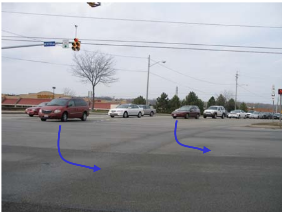
Southbound approach of SR306 showing the double left-turn lanes. A new pavement has recently been laid. Lane guide markings need to be placed.
