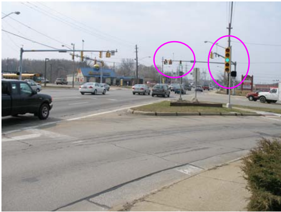
The pole-mounted signals, intended for the channelized right-turn lane, and the mast-mounted signals, intended for the through and left-turn lanes, operate in tandem causing the production of conflicting signal indications, shown in the photos below.
