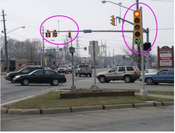
The pole-mounted signals, intended for the channelized right-turn lane, and the mast-mounted signals, intended for the through and left-turn lanes, operate in tandem causing the production of conflicting signal indications as shown in the photo. The signal heads mounted on the pole on the right of the road across the one shown in the photo display the same indications, hence the confusion.
