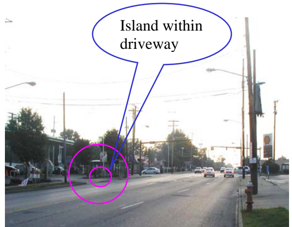
The 1 st driveway of the BP gas station, on Harvard Avenue, showing an island designed for right-in/right-out only traffic movements. See next photograph.
