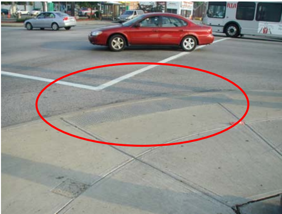
Truncated Domes on freshly laid concrete
