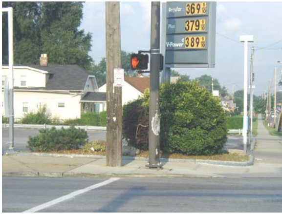
Sharp curvature, and objects within the lateral clearance area
