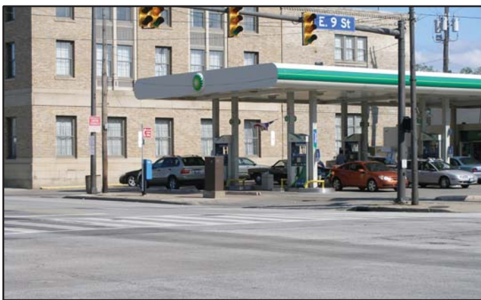
Picture 14: BP gas station, two driveways on Carnegie Avenue
