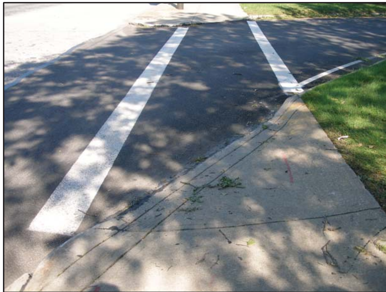
Picture 19: Curb ramps at the slip ramp on Carnegie Avenue eastbound approach
