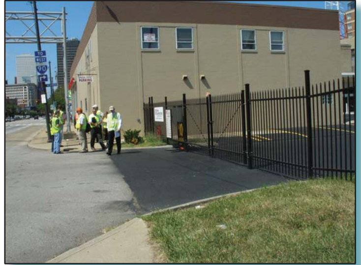
Picture 12: Missing crosswalk and edge lines markings
