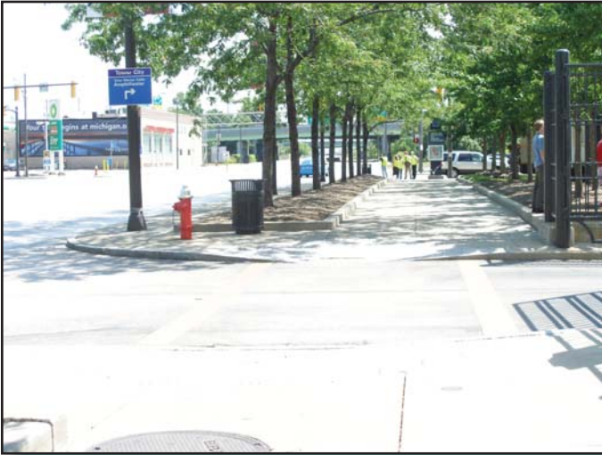
Picture 11: Crosswalk marking not in compliance with OMUTCD
