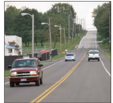
Munn Road was resurfaced from Stafford Road to Washington Street thanks to $200,000 in NOACA federal funding.
